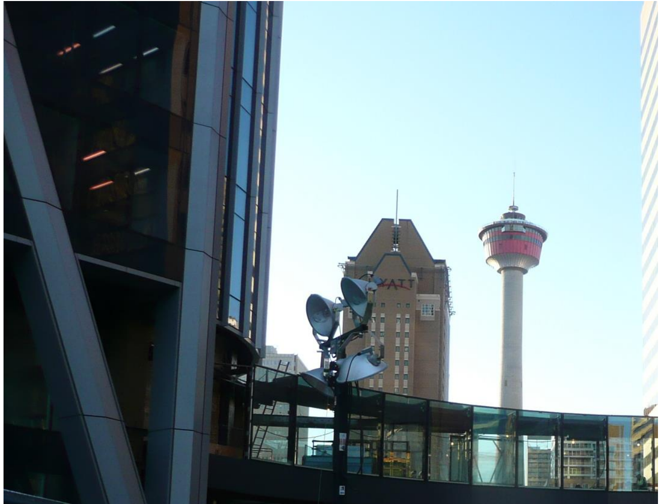
The Bow – Pedestrian Bridge, Calgary
