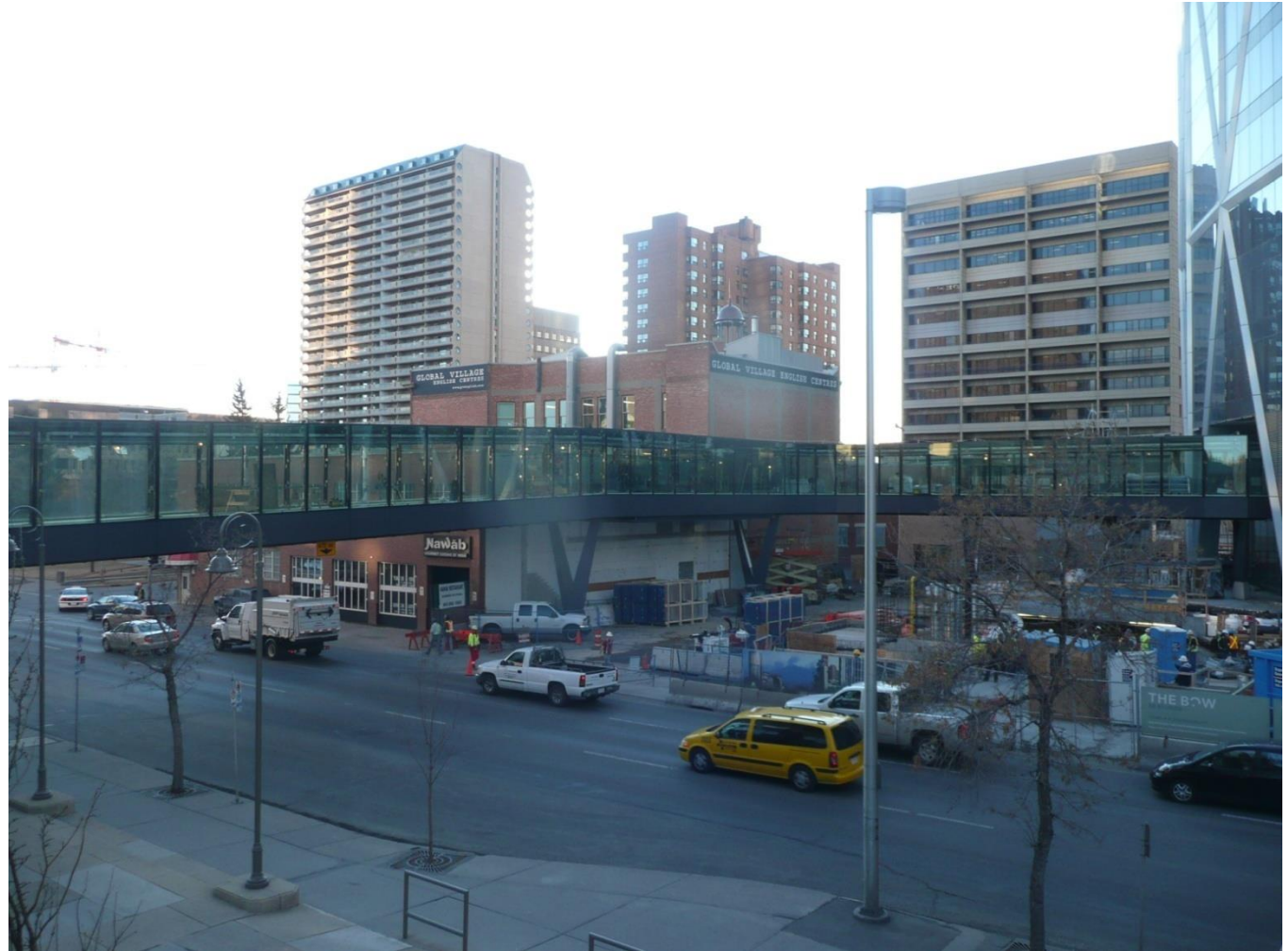
The Bow – Pedestrian Bridge, Calgary
