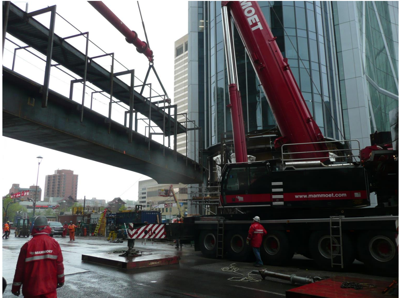
The Bow – Pedestrian Bridge, Calgary
