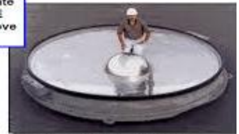
Concave Plate and Slider for FPS Bridge Bearing - Seismic retrofit of Benicia-Martinez Bridge, San Francisco, CA - 7.5 to 13 ft diameters - Displ. Capacity of 13 ft bearings = +/- 4.3 ft
