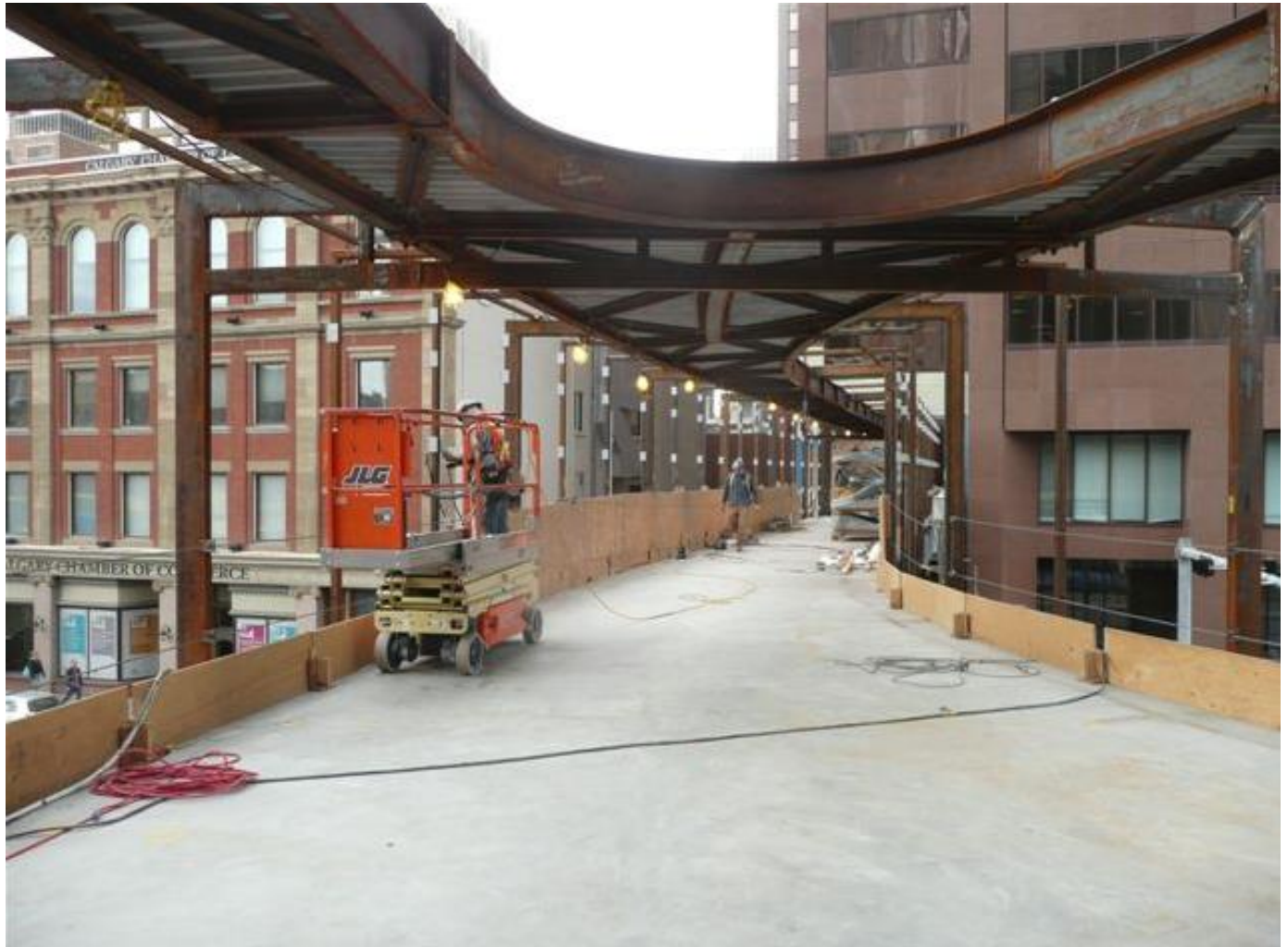
The Bow – Pedestrian Bridge, Calgary
