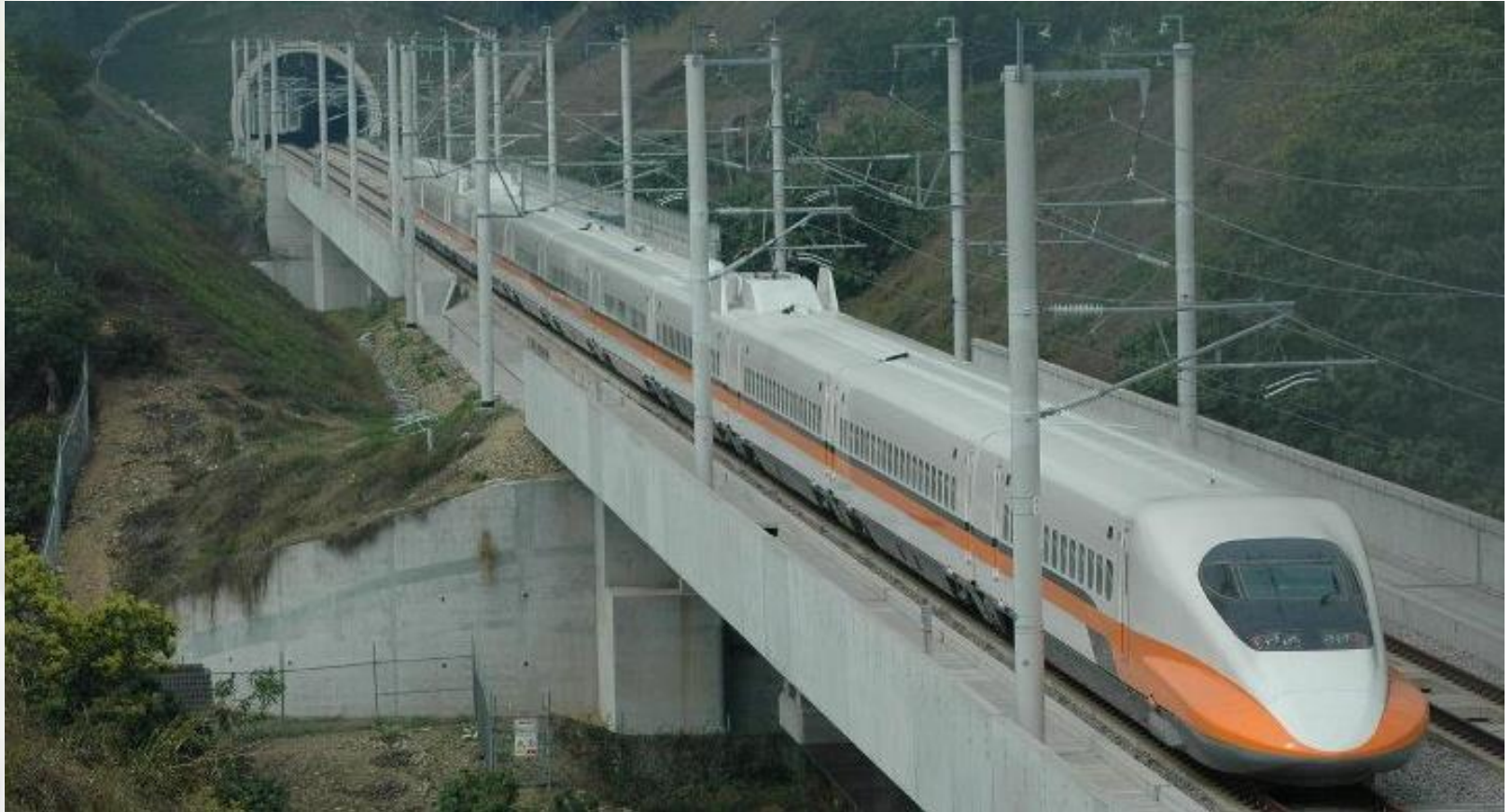
Taiwan High Speed Tunnel
